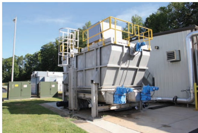
Dewatered sludge is conveyed into a seepex live bottom hopper buffer bin that holds 24 hours of product to ensure a consistent supply is sent to the dryer. The sludge cake is pushed through 80 feet of piping to the dryer.
